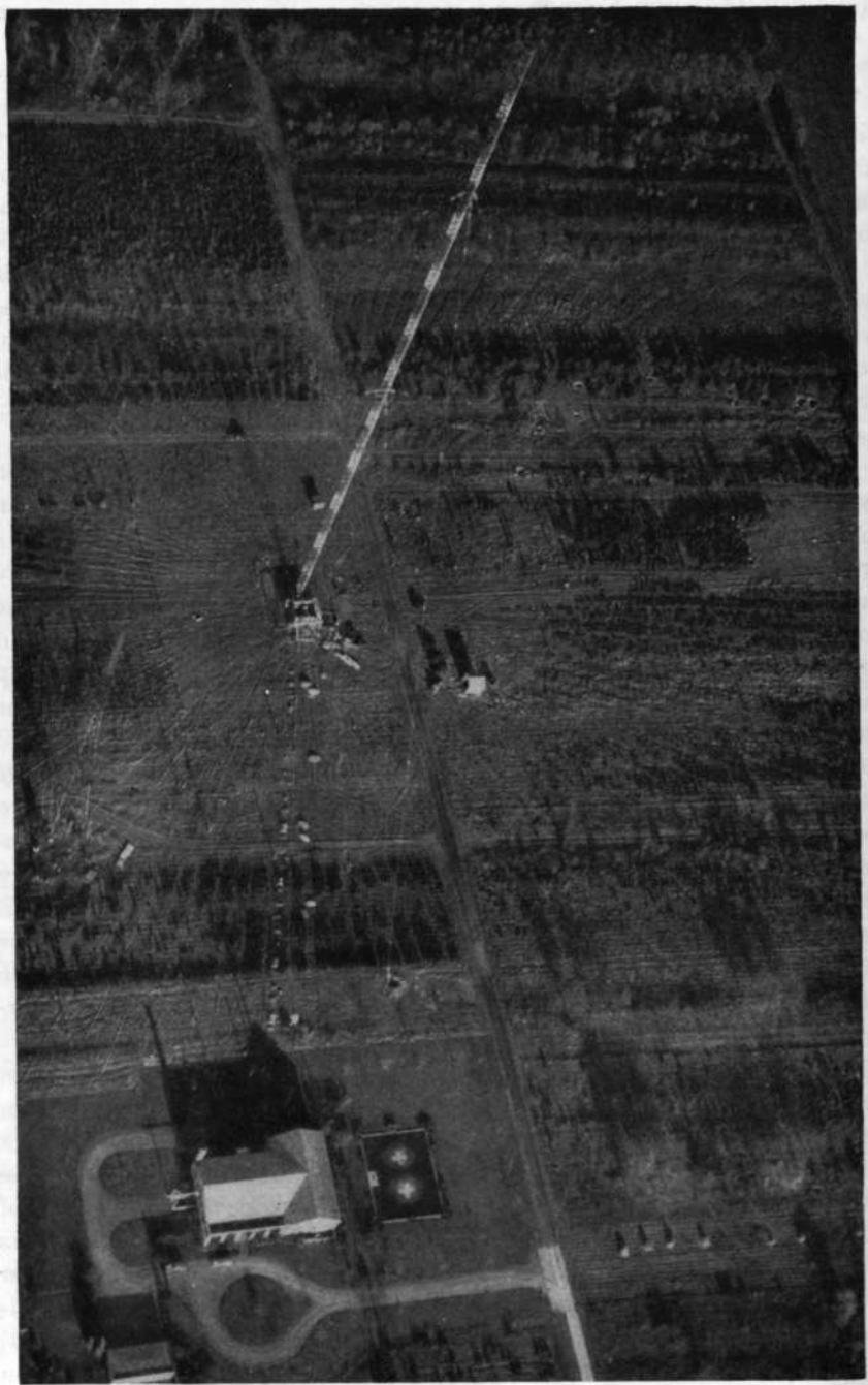
FIG. 2.52. Aerial view of a high-power broadcasting station (Radio Station WJZ when it was located at Bound Brook, New Jersey), showing the station building, the 750-foot radiator, and the freshly furrowed ground where the ground wires were plowed into the soil. (Photograph courtesy of National Broadcasting Company.)
