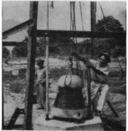
FIG. 2.62. The first step in the construction of a guyed vertical radiator for broadcasting—setting the base insulator. This photograph was taken in Peru. (Photograph courtesy of R. E. Lee.)
