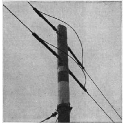
FIG. 4.101. Detail of a double-strain pole in a balanced two-wire feeder. (Photograph courtesy of Canadian Broadcasting Corporation.)
