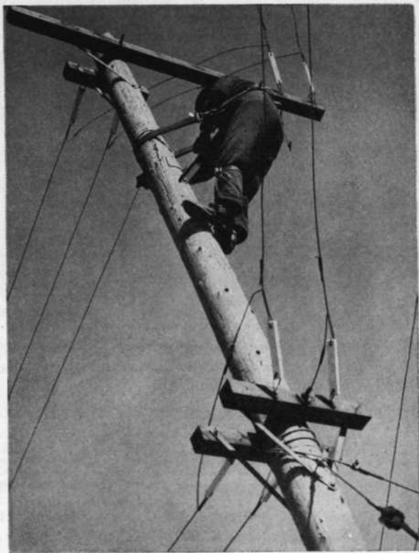
FIG. 4.83. Rigger working on a pole carrying balanced two-wire feeders for high-frequency broadcasting. This typifies many applications of this style of construction and hardware for broadcasting and communication use. This photograph was taken during construction, and the lines are not in final condition. Note the use of copper splicing sleeves at insulators, the attachment of guy wires, and crossarm hardware details. (Photograph courtesy of National Broadcasting Company.)
