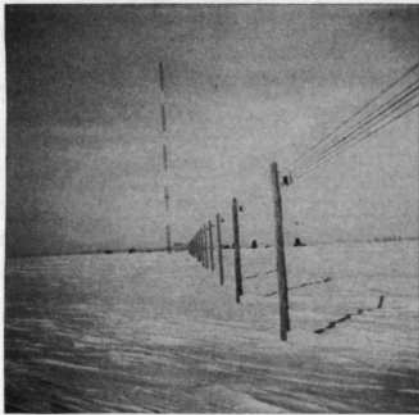
FIG. 4.71. A straight run of six-wire unbalanced (type XI) transmission line using the side-mounting bracket assembly on round wood poles. One radiator of a directive array with its coupling house, is in the distance. (Photograph courtesy of RCA Victor Company, Ltd., Montreal.)
