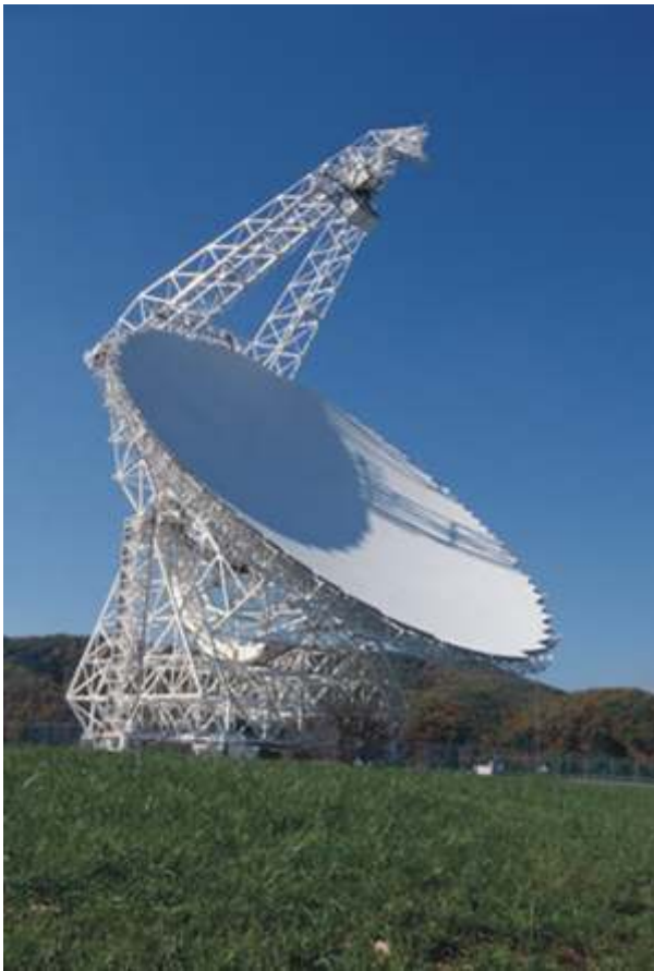
Green Bank 100m Antenna
